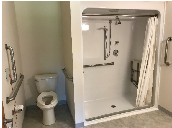
Living unit bathroom accessibility features
