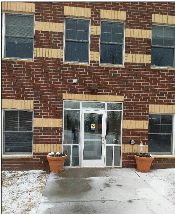
Dedicated entrance to Boutwells Landing ADS
