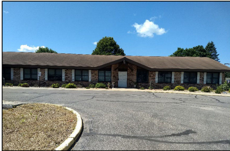
Building wing that contains the Care Center Apartments
