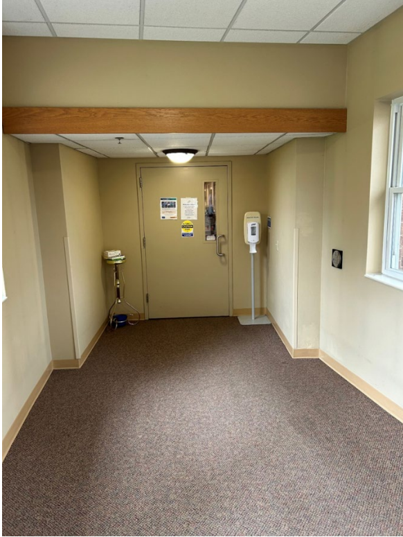
Hallway and door connecting SNF to HCBS setting.
