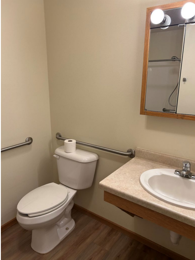
Grab bars by toilets in every bathroom with wheelchair accessible sink.
