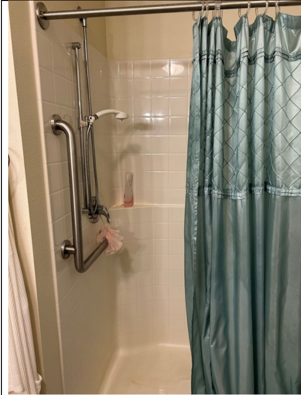
Grab bars and handheld shower head on shower wall. Shower seat behind the shower curtain.
