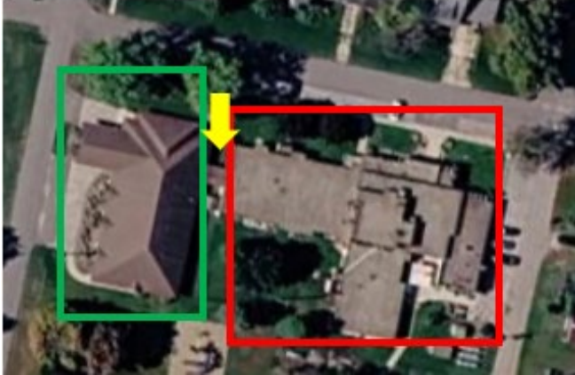
Aerial view of Ostrander indicating connection between buildings
