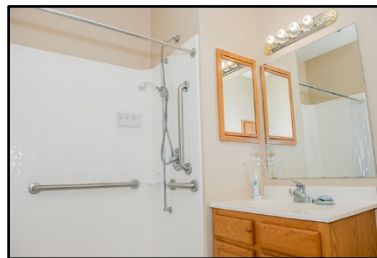
Accessible shower with grab bars
