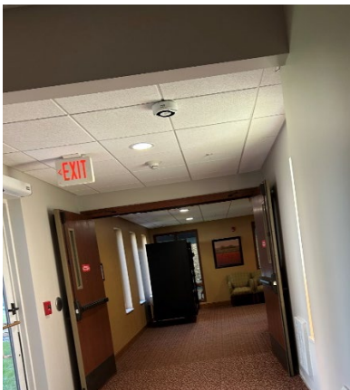
Connection number one to nursing facility
