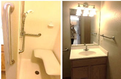
Grab bars and shower bench
